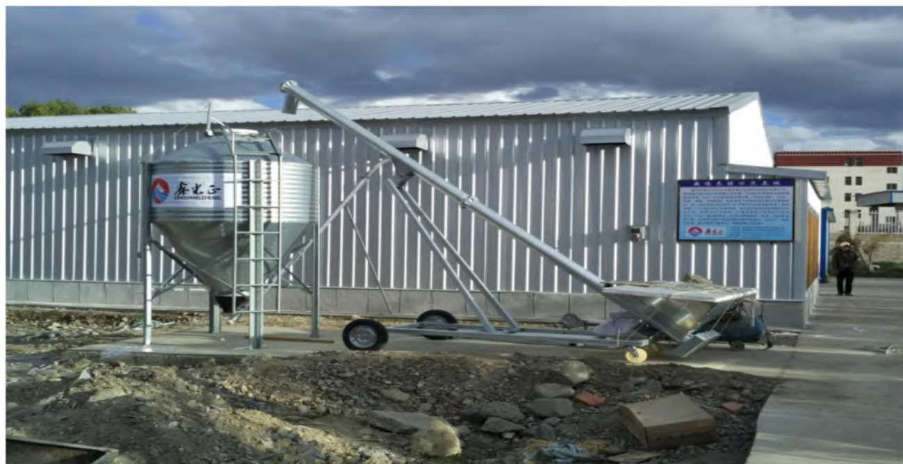
鸡舍外观 House Appearance
