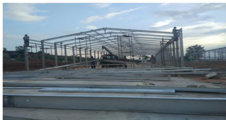
C型钢结构鸡舍 C Type Rigid Structure Chicken House
