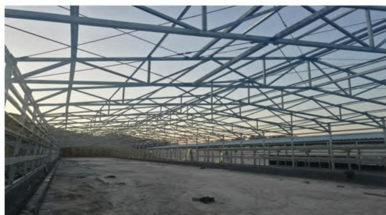
桁架结构鸡舍 Truss Structure Chicken House
