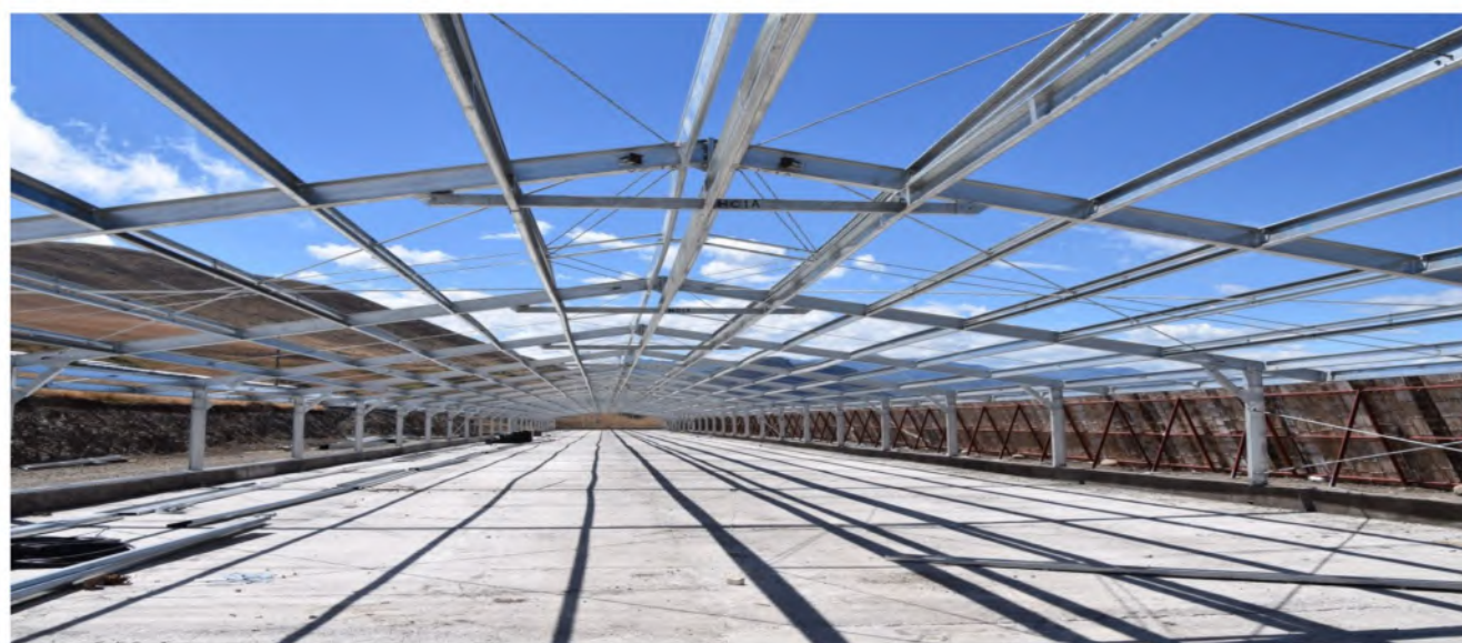
菲律宾平养肉鸡舍 Philippine Ground Raising Broiler House
